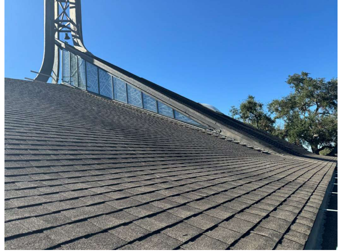
Photograph 5. Overview of the north upper clerestory windows at St. Andrew's.
