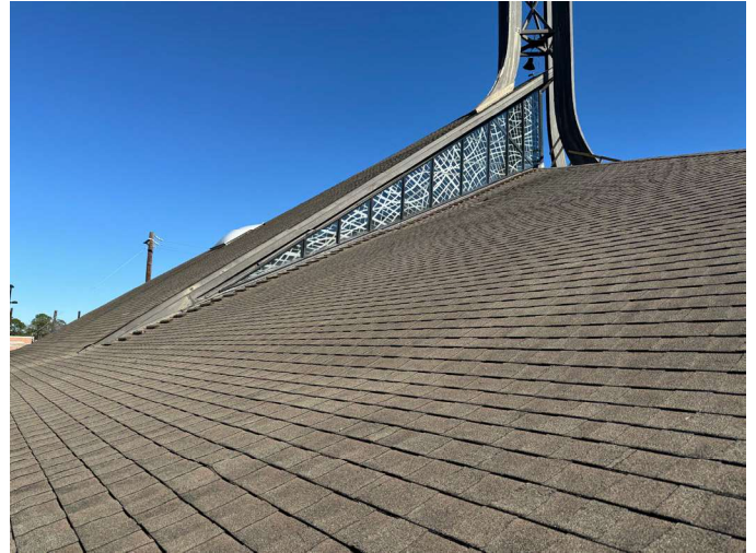
Photograph 8. Overview of the west upper clerestory window at St. Andrew's.
